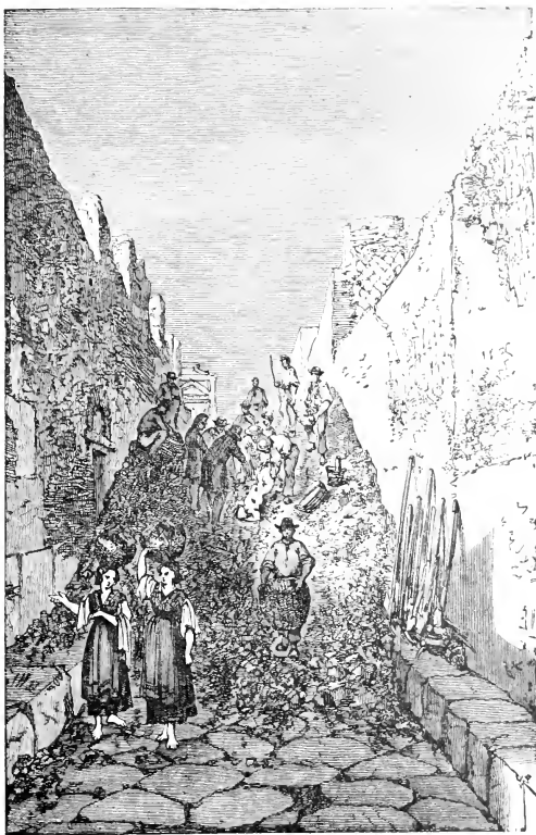
CLEARING OUT A NARROW STREET IN POMPEII.
